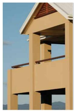
5 It is important to monitor areas that are heavily exposed to the elements such as parapets and balcony handrail tops. Due to the minimal slope on these areas it will tend to hold dirt and grime which can potentially lead to mould over time if not regularly washed. These building sections should also be checked for any movement over time due to the extremes of thermal movement so it is critical that they are inspected and maintained.
