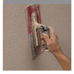
Recoating is recommended after a minimum of 7 to 10 years to rejuvenate the surface appearance. This can be done by using *Dulux AcraTex* elastomeric top coat protective membrane to a selected *Dulux AcraTex* colour which will protect from air pollutants, water ingress and dirt accumulation to provide a new low maintenance surface.
